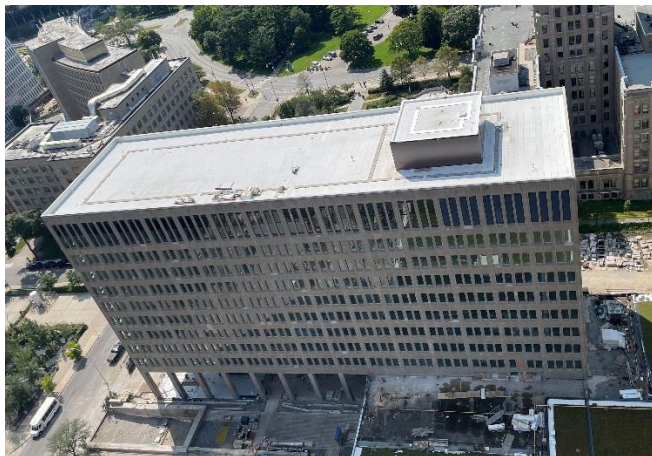
Pictured: 'Punch window' installation is completed.
