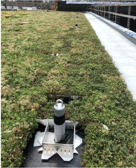
Photo: New podium green roof
