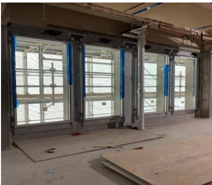
Photo: New windows in Ferguson
