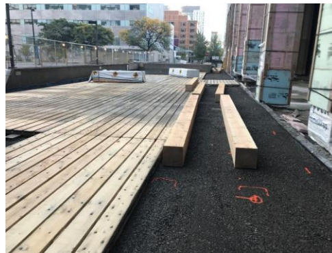
Photo: Mud mats protect heritage elements beneath the scaffolding.
