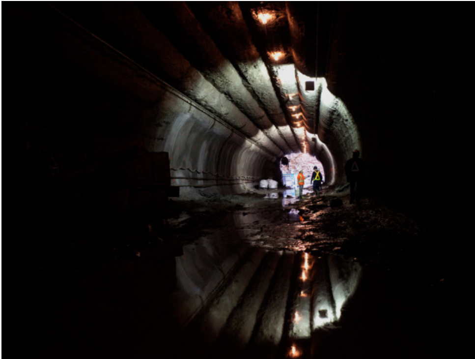
Construction of the Billy Bishop Tunnel in Toronto in October, 2013, a successful P3 infrastructure initiative.
