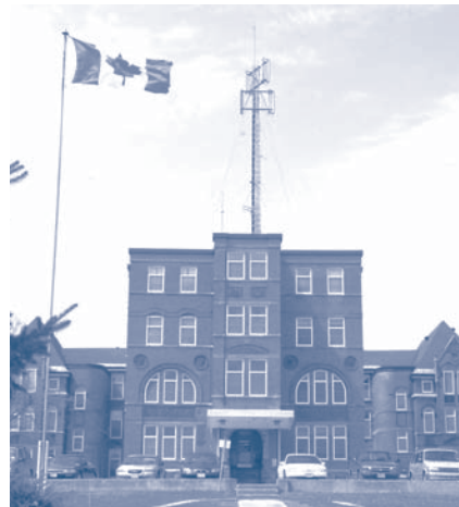
St. Lawrence Valley Treatment Centre, Brockville
