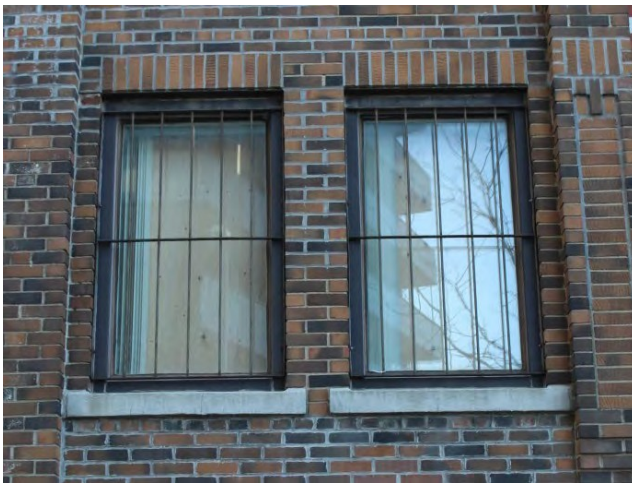
Figure 45: Typical Window Replacement – North Elevation - Ground Floor Credit: SBA, November 2020
