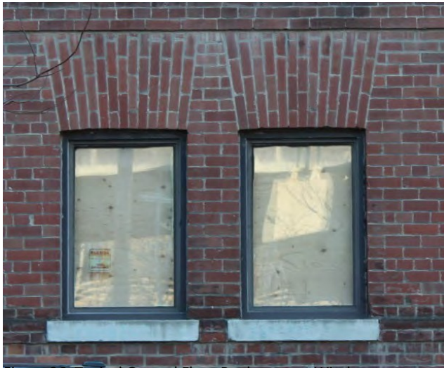
Figure 36: Typical Ground Floor Replacement Window Credit: SBA, November 2020
