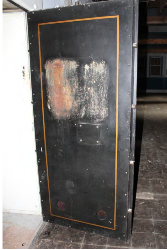
Figure 57: Ground Floor Vault Door 2 – Interior Credit: SBA, November 2020
