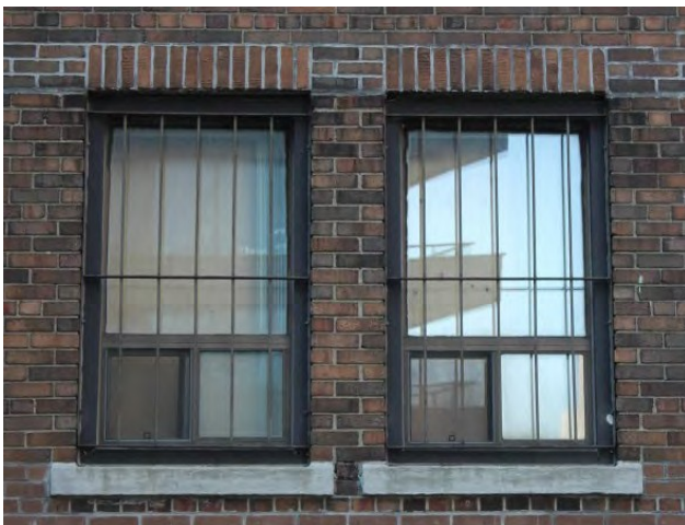
Figure 47: Typical Window Replacement – East and South Elevations Credit: SBA, November 2020
