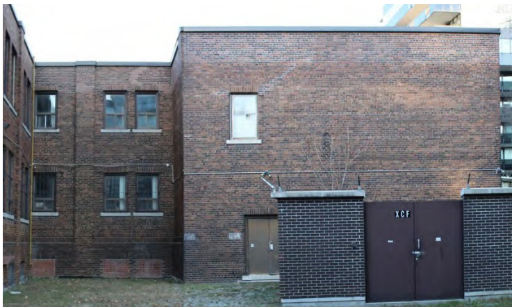
Figure 42: 171 Eastern Avenue – Office – South (Rear) Elevation Credit: SBA, November 2020
