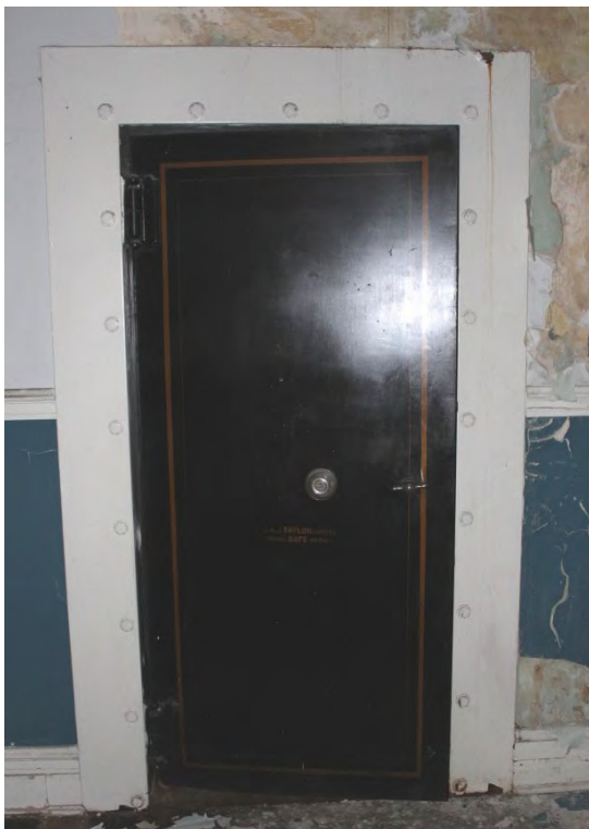
Figure 54: Ground Floor Vault Door 1 - Exterior Credit: SBA, November 2020
