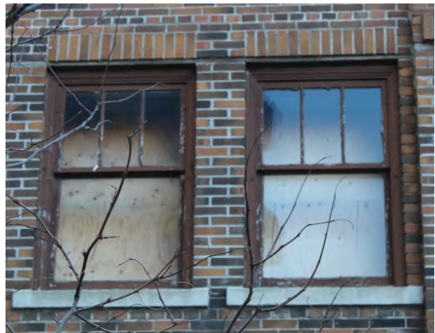
Figure 46: Original Windows - North Elevation – Second Floor Credit: SBA, November 2020
