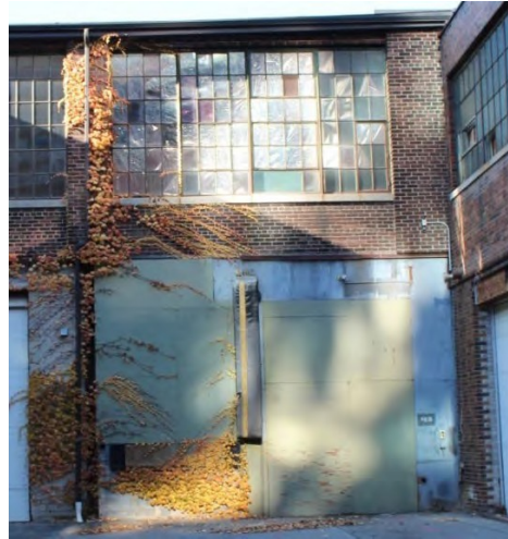
Figure 33: 169 Eastern Avenue – Warehouse – East (Side) Elevation Credit: SBA, November 2020
