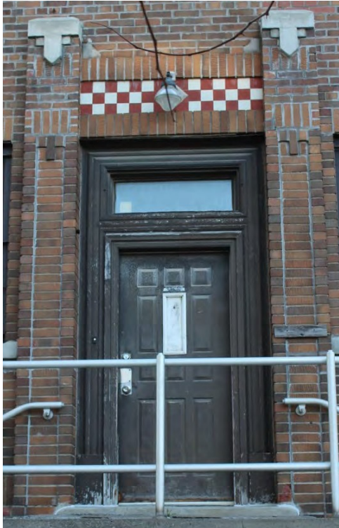
Figure 49: Front Entrance on Eastern Avenue Credit: SBA, November 2020
