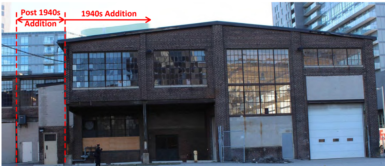
Figure 64: 185 Eastern Avenue – 1935 Machine Shop 1940s Addition and Post 1940s Addition – West Elevation Credit: SBA, November 2020
