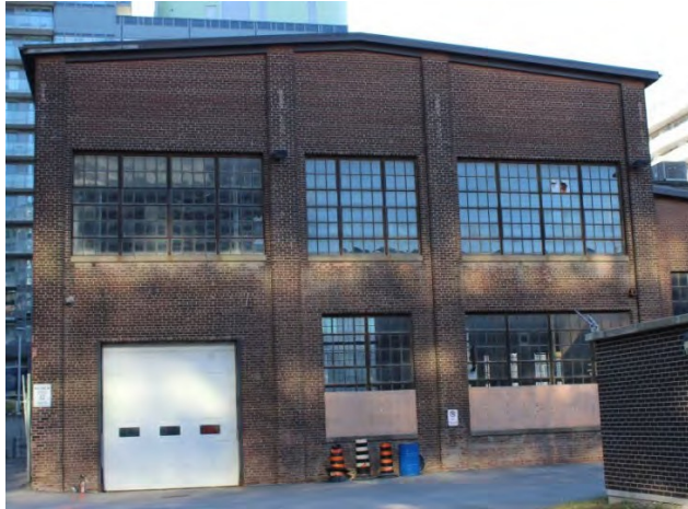
Figure 66: 185 Eastern Avenue – 1939 Machine Shop – North Elevation Credit: SBA, November 2020
