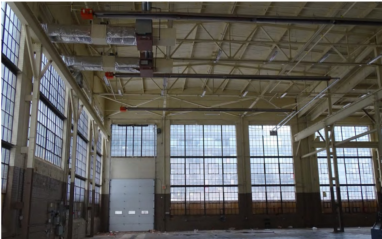
Figure 76: 1939 Machine Shop showing equipment structure Credit: SBA, November 2020
