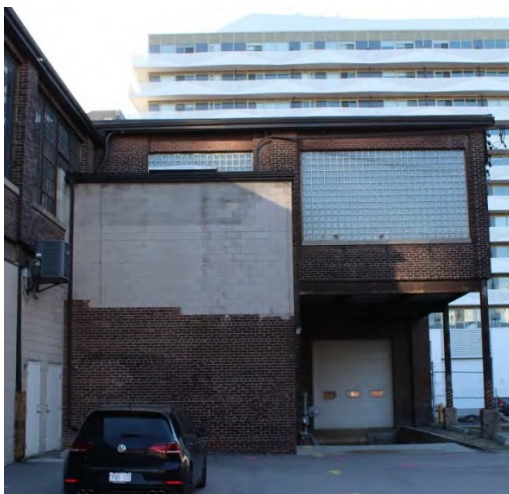
Figure 65: 185 Eastern Avenue – 1935 Machine Shop 1940s Addition –North Elevation Credit: SBA, November 2020
