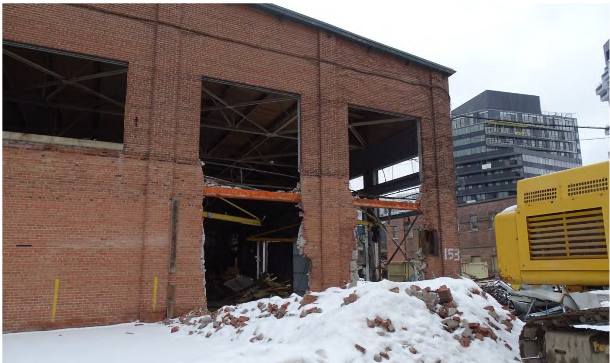
Figure 23: South (Rear) Elevation: Post Partial Demolition Credit: SBA, February 2021
