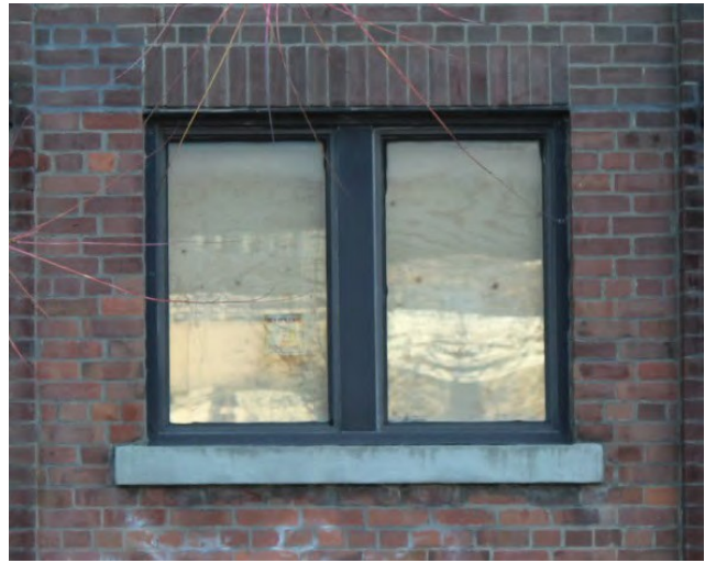
Figure 35: Window Replacement at Original Entrance Location Credit: SBA, November 2020
