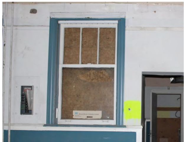
Figure 48: Original window located internally Credit: SBA, November 2020
