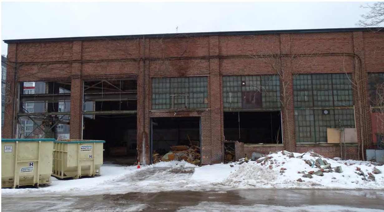
Figure 21 East (Side) Elevation: Post Partial Demolition Credit: SBA, February 2021
