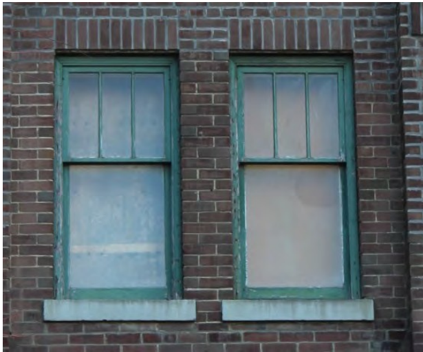
Figure 34: Original Window Type – Second Floor Credit: SBA, November 2020
