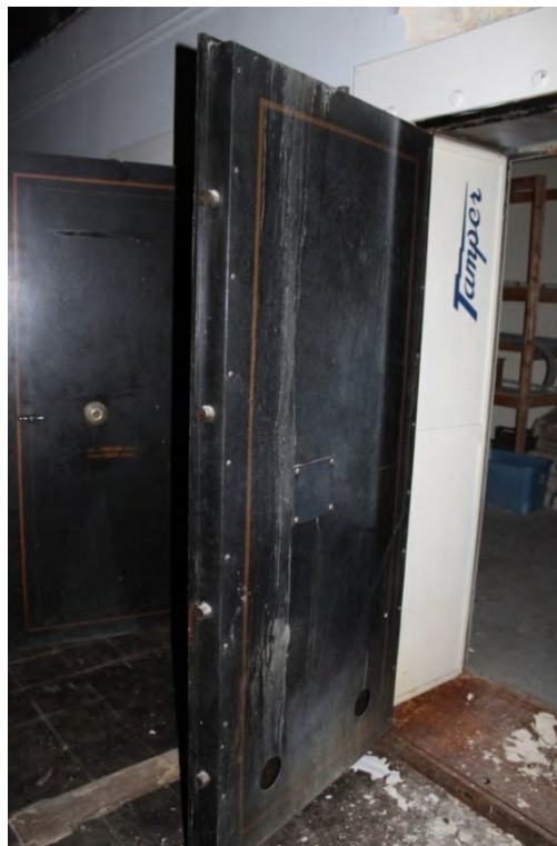
Figure 55: Ground Floor Vault Door 1 – Interior Credit: SBA, November 2020
