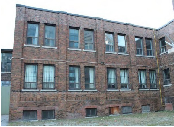
Figure 43: 171 Eastern Avenue – Office Post 1941 Addition – East (Side) Elevation Credit: SBA, November 2020
