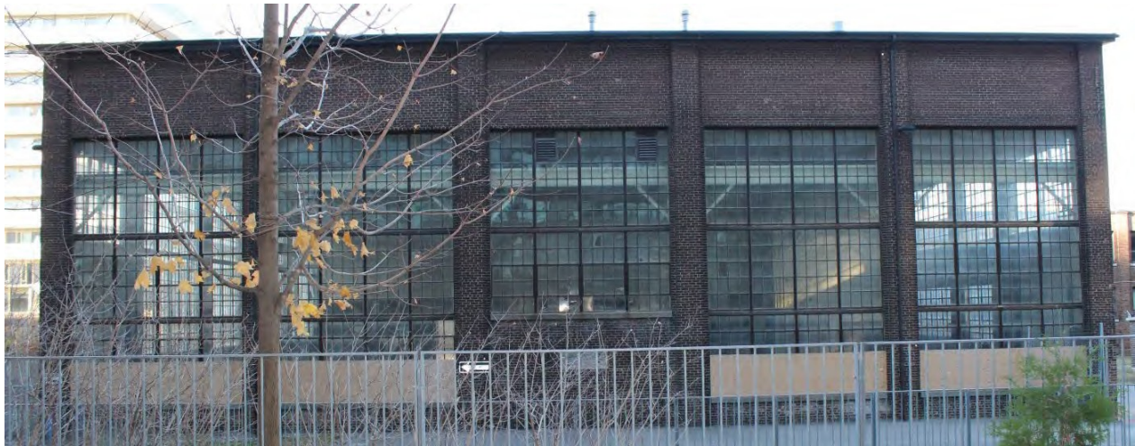
Figure 68: 185 Eastern Avenue – 1939 Machine Shop – East Elevation Credit: SBA, November 2020
