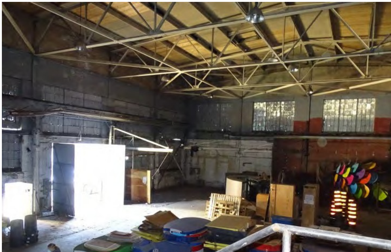
Figure 26: Interior View of Cleaning Room looking Southeast from Mezzanine Credit: SBA, November 2020
