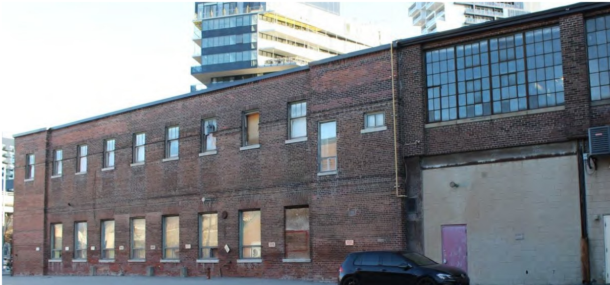
Figure 31: 169 Eastern Avenue – Warehouse – West (Side) Elevation Credit: SBA, November 2020
