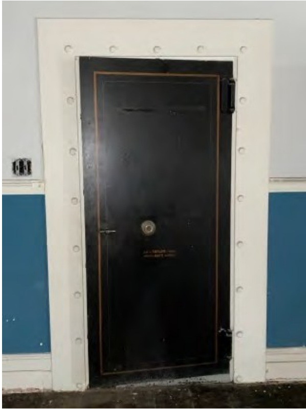
Figure 56: Ground Floor Vault Door 2 –Exterior Credit: SBA, November 2020
