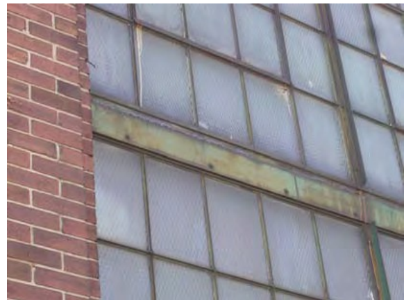
Figure 24: Exterior detail at steel angle. Credit: Commonwealth, 2010.
