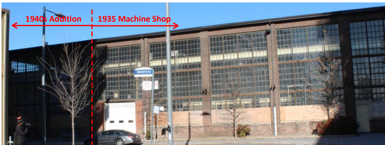
Figure 62: 185 Eastern Avenue – 1935 Machine Shop and 1940s Addition – South Elevation Credit: SBA, November 2020
