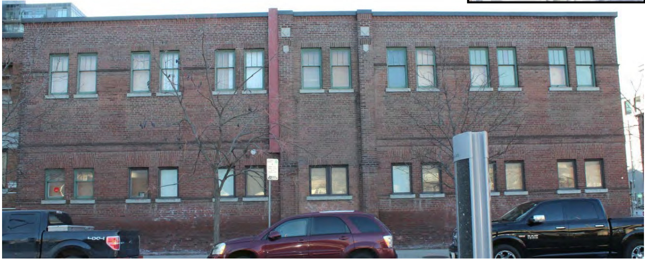
Figure 30: 169 Eastern Avenue – Warehouse – North (Front) Elevation Credit: SBA, November 2020
