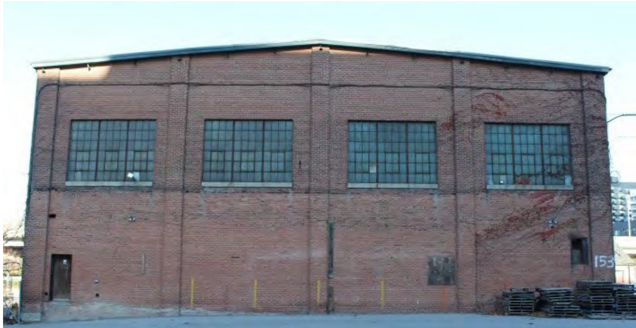
Figure 22: South (Rear) Elevation: Prior to Partial Demolition Credit: SBA, November 2020
