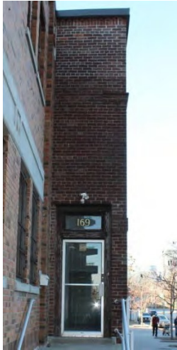
Figure 32:169 Eastern Avenue – Warehouse – East (Side) Elevation Credit: SBA, November 2020
